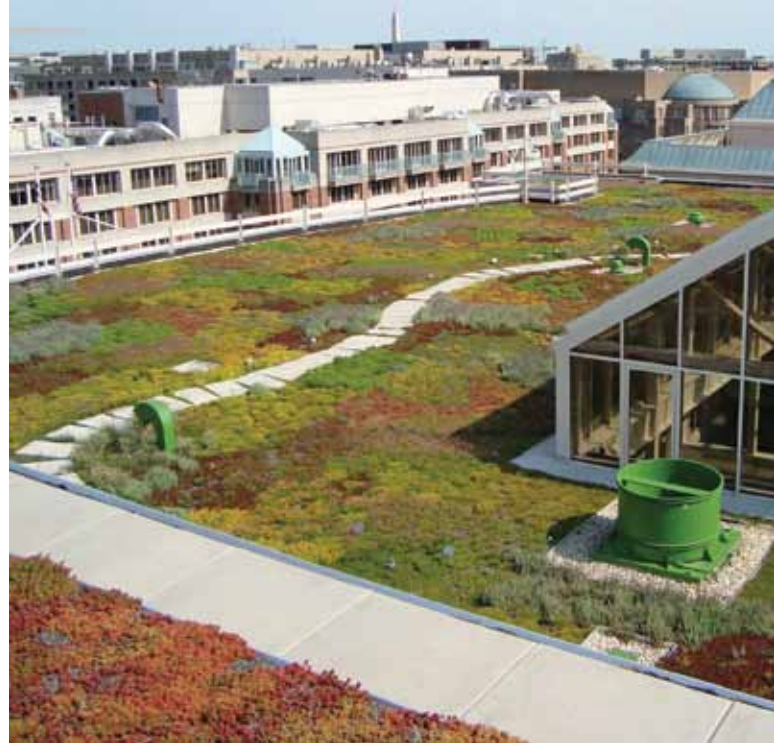
Green roof on the headquarters building of the World Wide Fund for Nature in Washington DC
