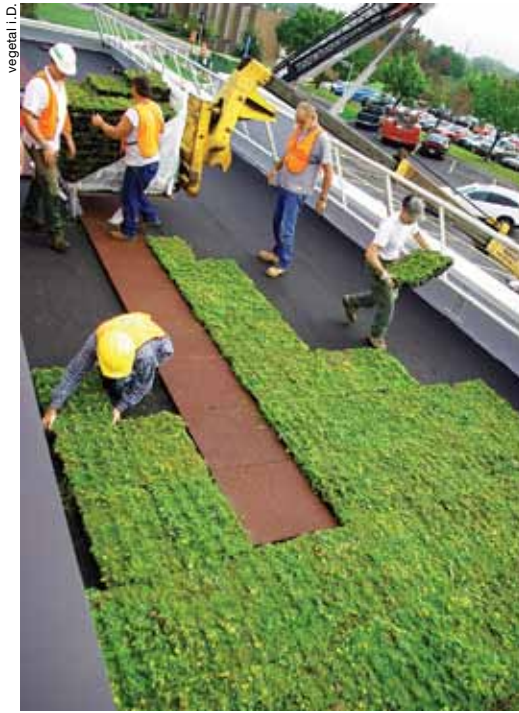
Installing Hydropack green roof trays on a Shenandoah University rooftop
