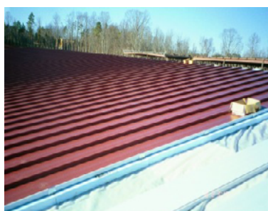
Figure 4: Standing Seam Metal Roofing (SSMR) Assemblies
