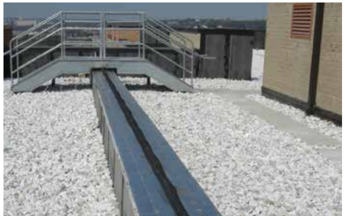
Prefabricated expansion joint
