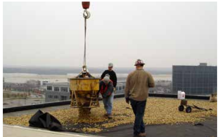
Stone ballast installed
