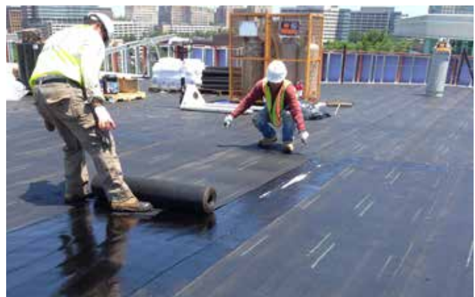
Protection layer installed
