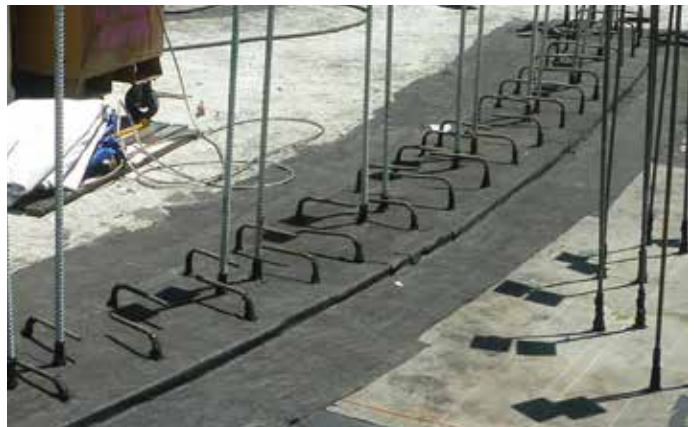
Through wall curb detailing
