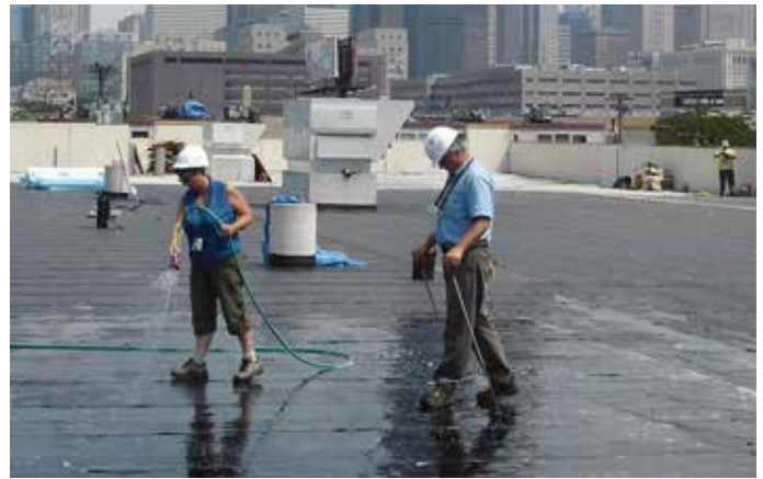
Electric conductivity testing
