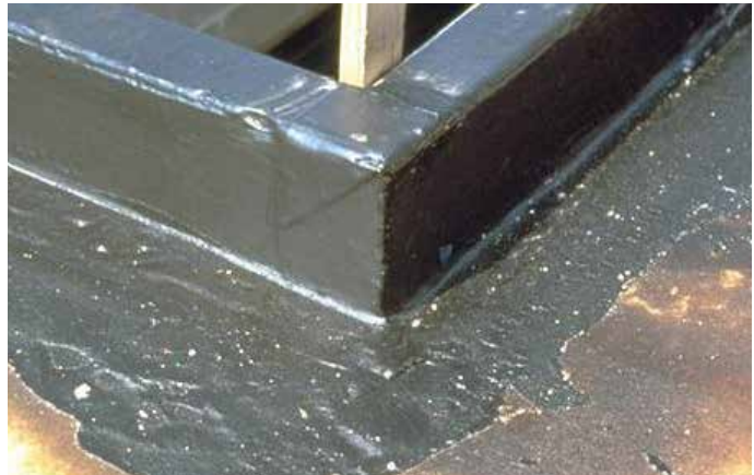
Curb flashing installed
