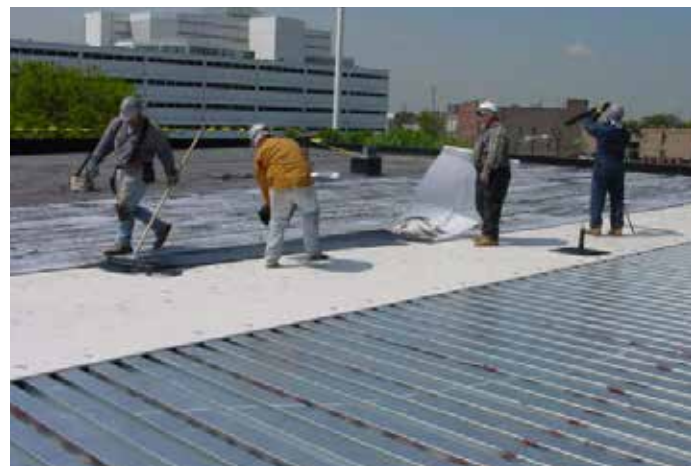
USG Securock Over Metal Deck Substrate
