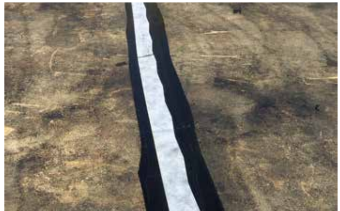
Cold or control joints
