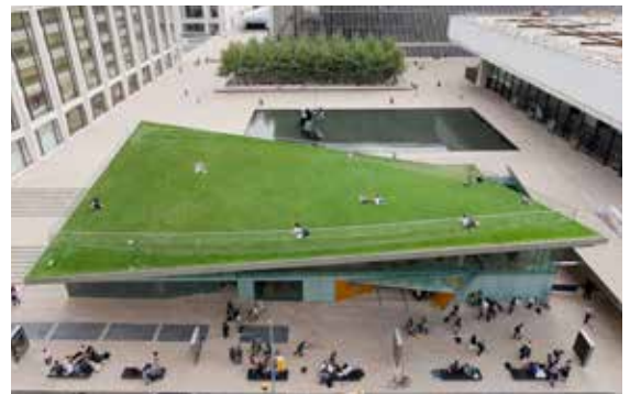
Hypar Pavilion at Lincoln Center - New York, NY
