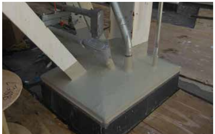
HydroSeal PMMA flashing
