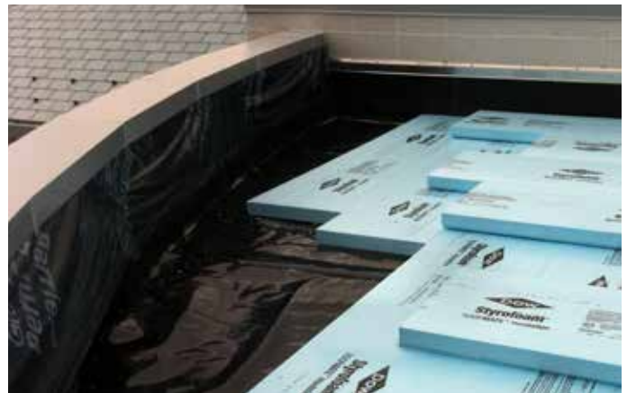
STYROFOAM™ Insulation installed
